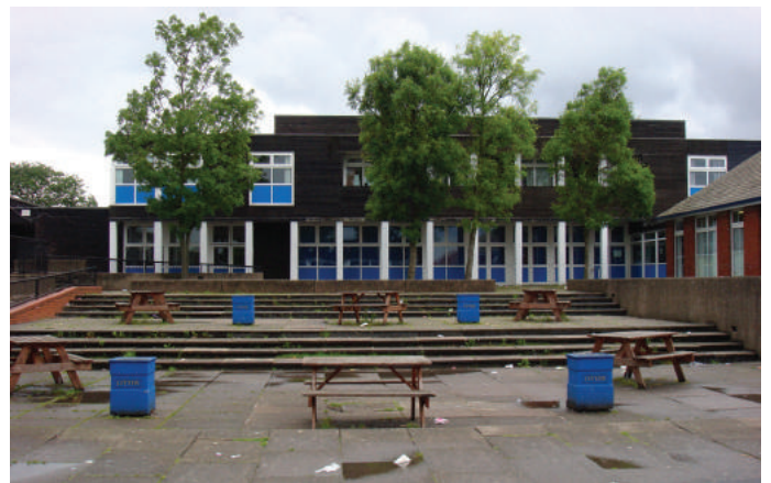
Existing school playground
