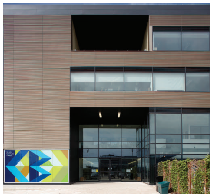
Kirk Balk Community College entrance with lightbox
