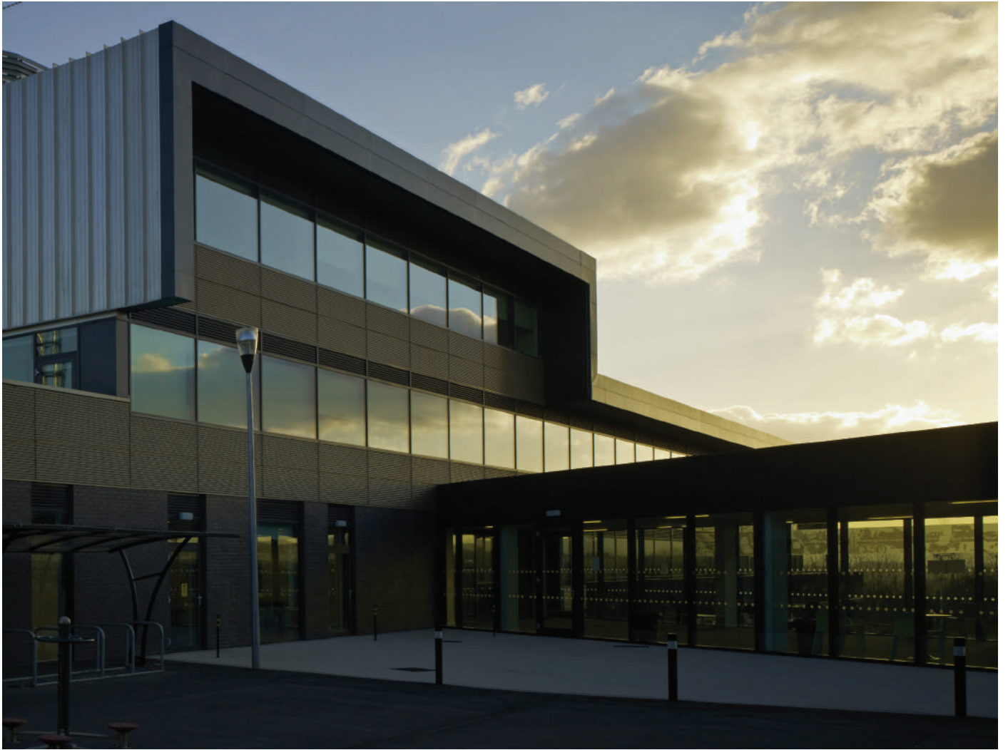
View of the main building's folding roofscape
