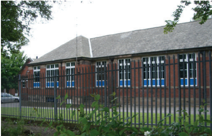
Existing School buildings to Kirk Balk Street
