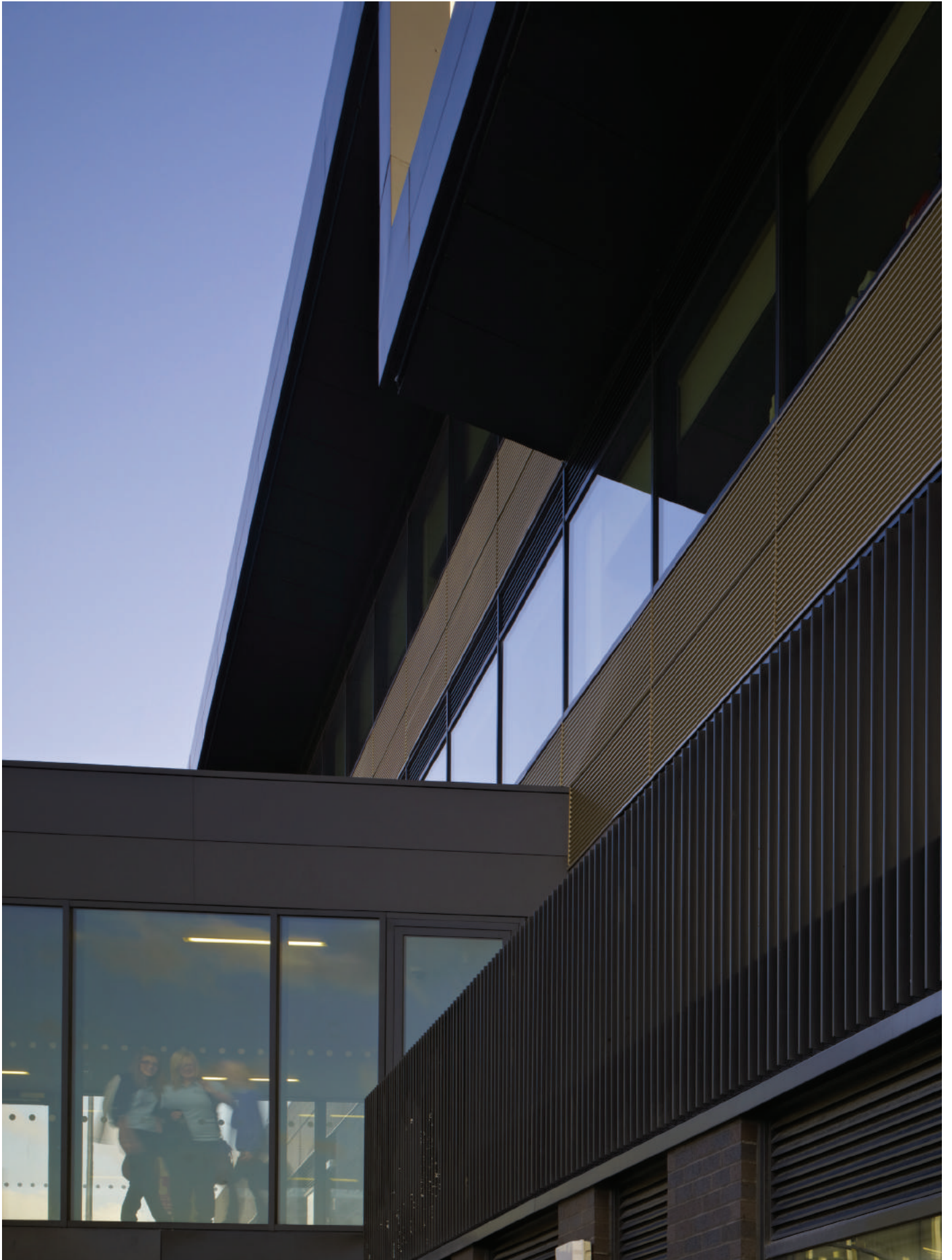
Detail view of the Main Building façade
