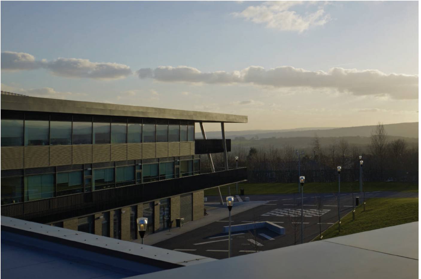
View of the Main Building's strong horizontal emphasis, accentuated by dark grey ribbon windows
