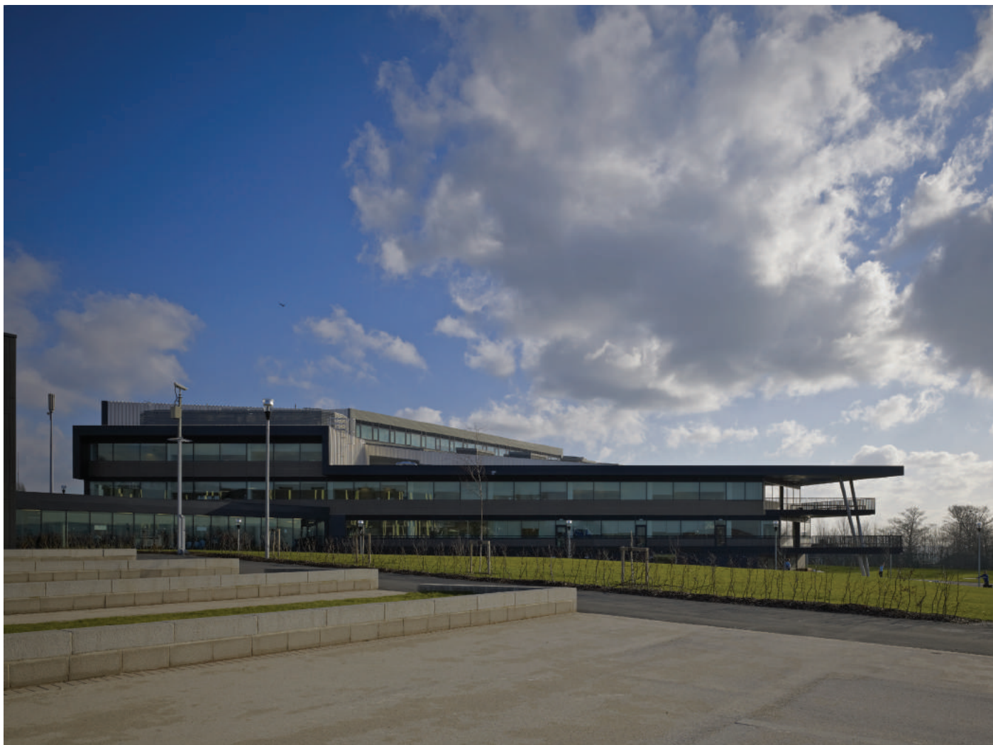
View of the Main Building's folding roofscape as the building steps down the slope
